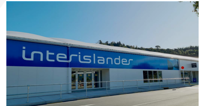
New builds and offsite prefab manufacturing
