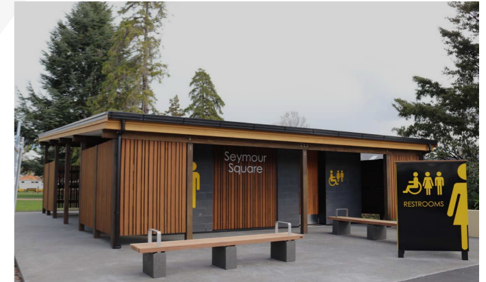
Marlborough District Council Seymour Square restrooms $567K
