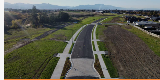
Bulk earthworks and subdivisions
