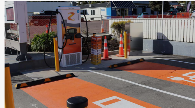
EV charger installation
