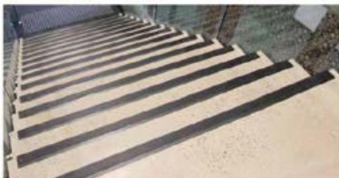
**Depth of the riser:** Where the luminance contrast strip extends down the front of the stair, the strip cannot be more than 10mm. This limitation is to avoid confusing the location of the leading edge of the tread. If the front of the nosing body is not a contrast or "blends in", and it is clearly differentiated from the luminance contrast strip, then the stair nosing body can extend any distance down the riser.
